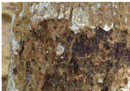
Figure 22: damage characteristic of Amitermes observed after removing Odontotermes plaster, a few traces of which can be seen to the left of the photo.
